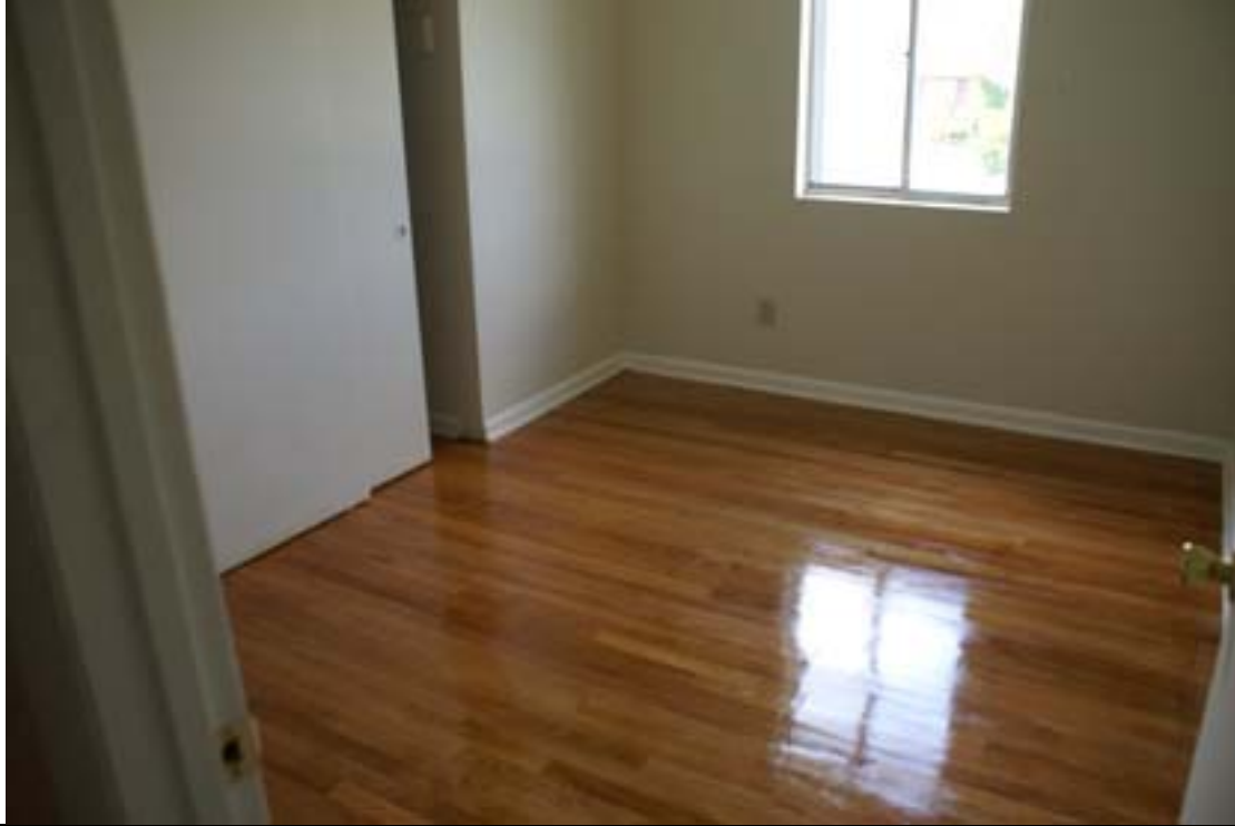
2716 Bertrand Rd Bedroom #1 floor after Renovation
