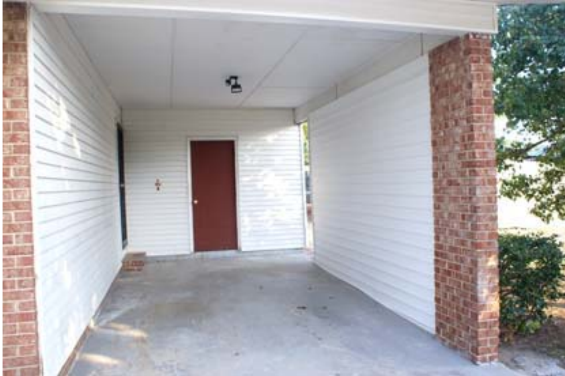
2716 Bertrand Rd Garage after Renovation
