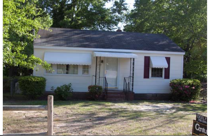
Front of House Renovated
