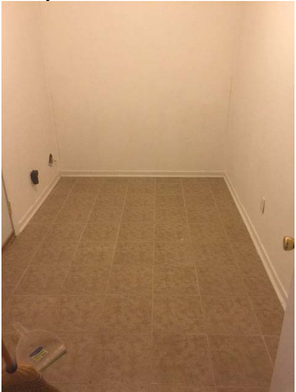
Laundry Room Renovated
